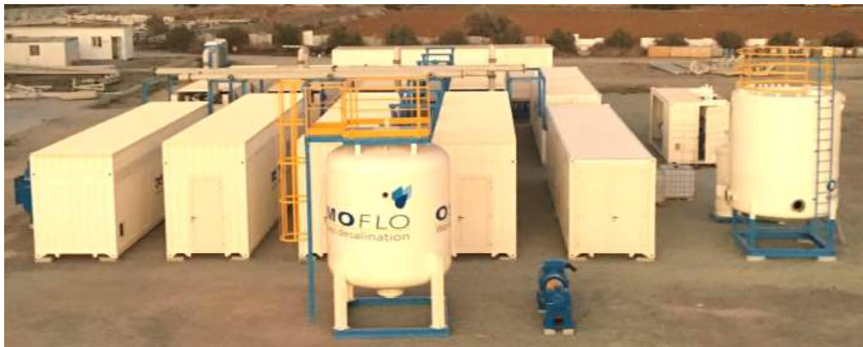
Figure C-18. Osmoflo Containerized 1.8-mgd Desalination System
