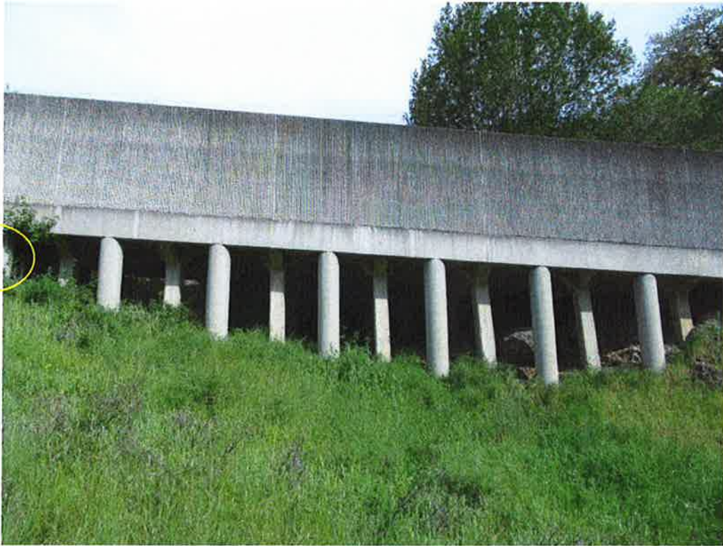
The raised portion of the spillway, above, and the extensometers monitoring movement along a crack through the spillway foundation, below. The location of the instrumentation is circled in the top photograph.
