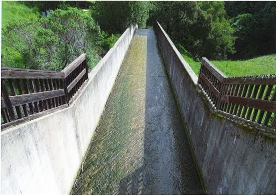
Looking down the raised spillway section, above. The spillway channel outfall and the outlet box are shown below.
