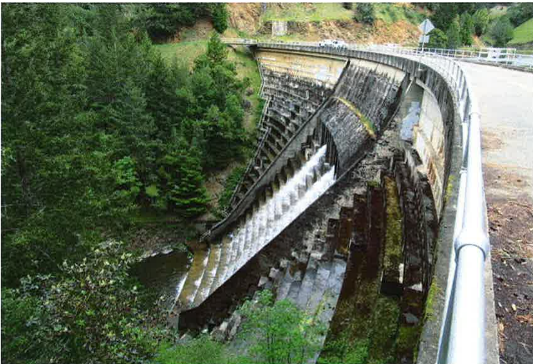
The downstream face as viewed from the left abutment.
