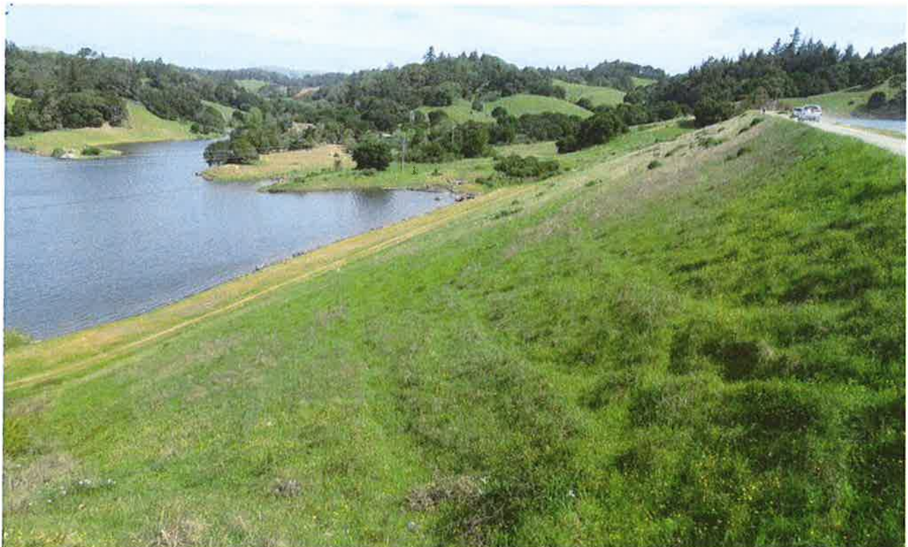
The downstream face as viewed from the right abutment, above, and the left abutment, below. Vegetation control remains generally quite good.
