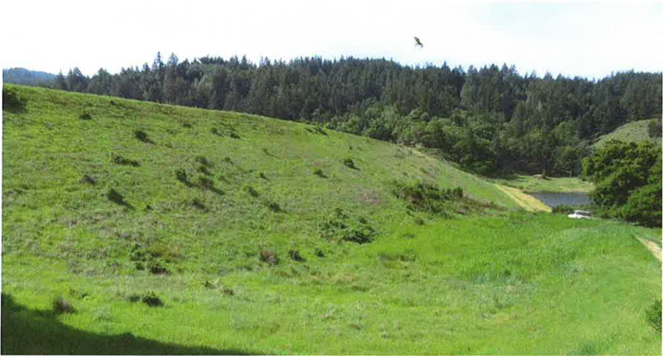
The downstream face as viewed from the right abutment, above, and the left abutment, below. Vegetation control remains generally quite good.
