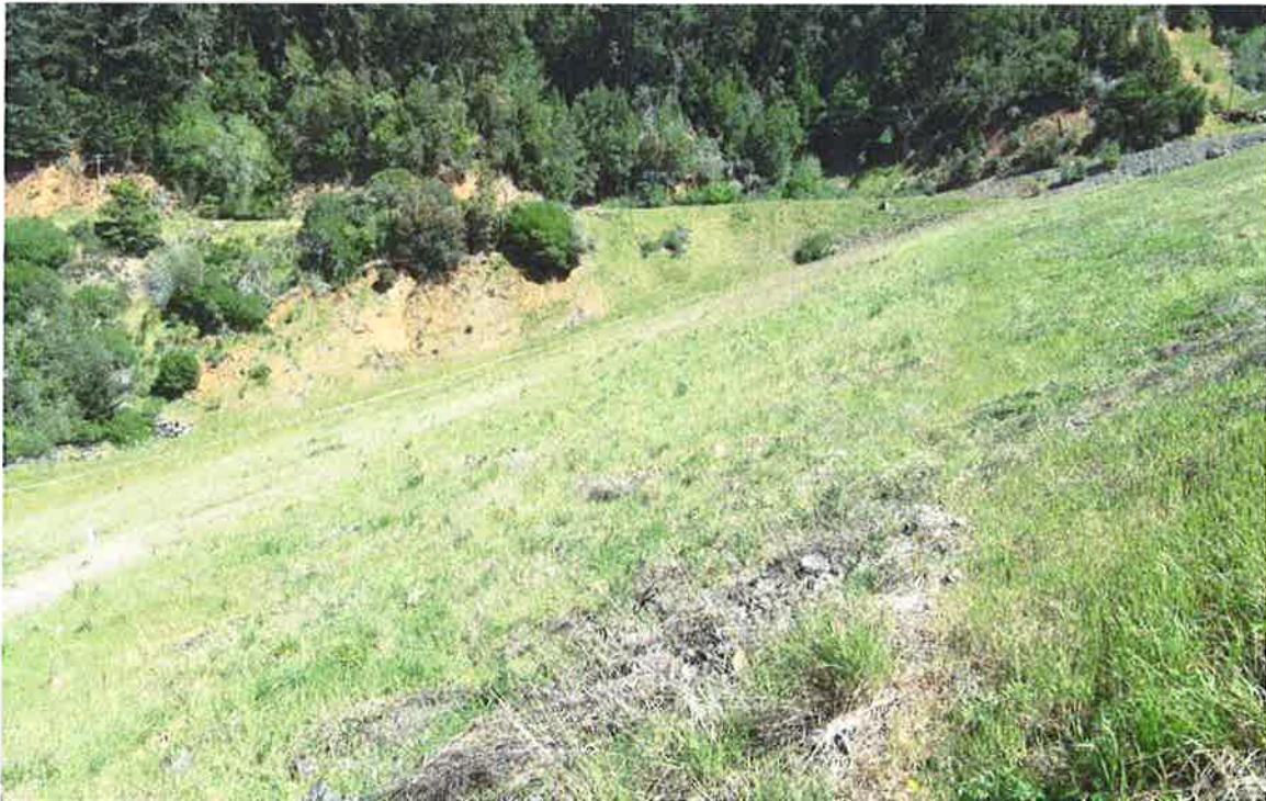
The downstream face as viewed from the right abutment, above, and from the left abutment, below. As is evident from the photographs, vegetation control is now excellent.
