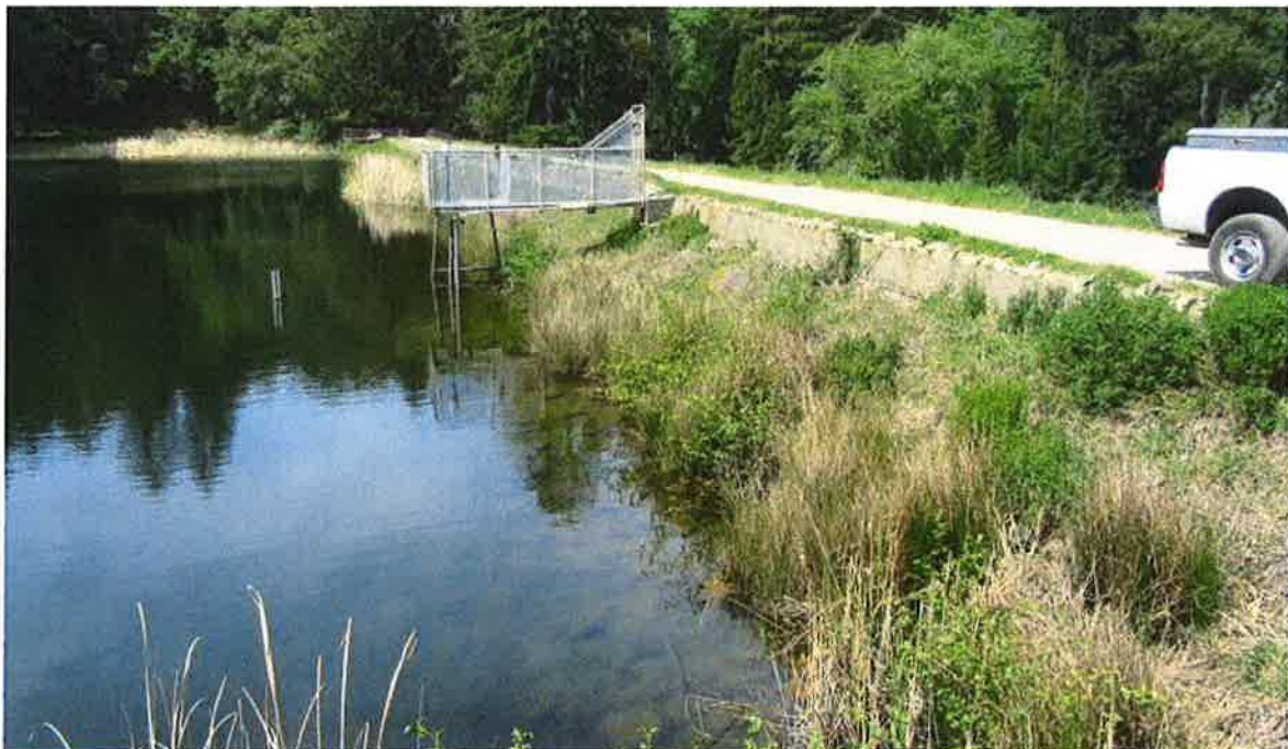
The upstream face as viewed from the left abutment, above, and as viewed from the right abutment, below. Vegetation control along the upstream face needs improvement, and numerous small trees, bushes, and other woody vegetation that have accumulated along the waterline and upstream groins require removal.
