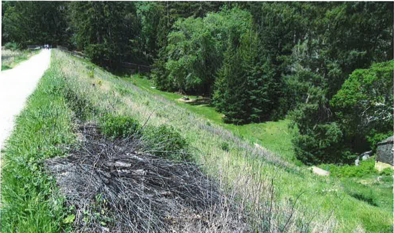
The downstream face as viewed from the left abutment, above, and as viewed from the right abutment, below. Vegetation control along the downstream face is satisfactory, and access for inspection and monitoring is good.
