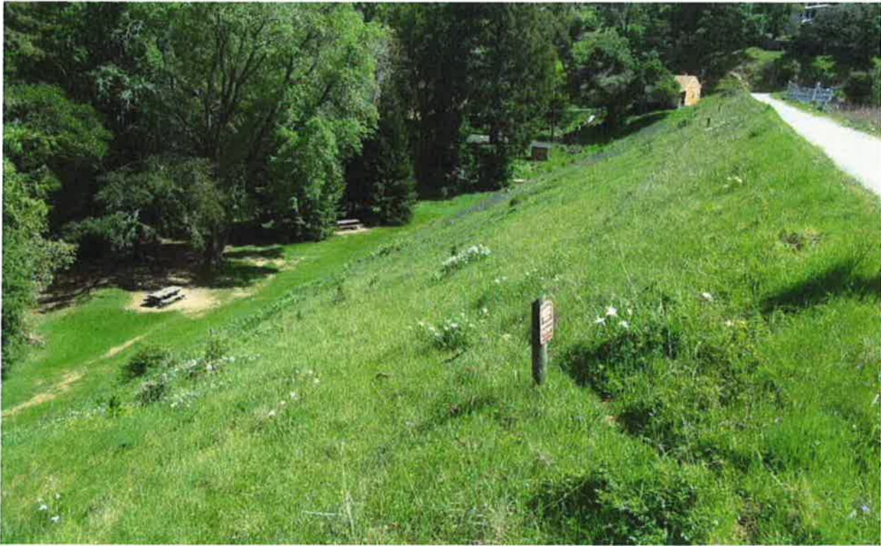
The downstream face as viewed from the left abutment, above, and as viewed from the right abutment, below. Vegetation control along the downstream face is satisfactory, and access for inspection and monitoring is good.
