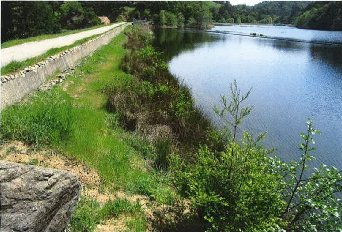
The upstream face as viewed from the left abutment, above, and as viewed from the right abutment, below. Vegetation control along the upstream face needs improvement, and numerous small trees, bushes, and other woody vegetation that have accumulated along the waterline and upstream groins require removal.
