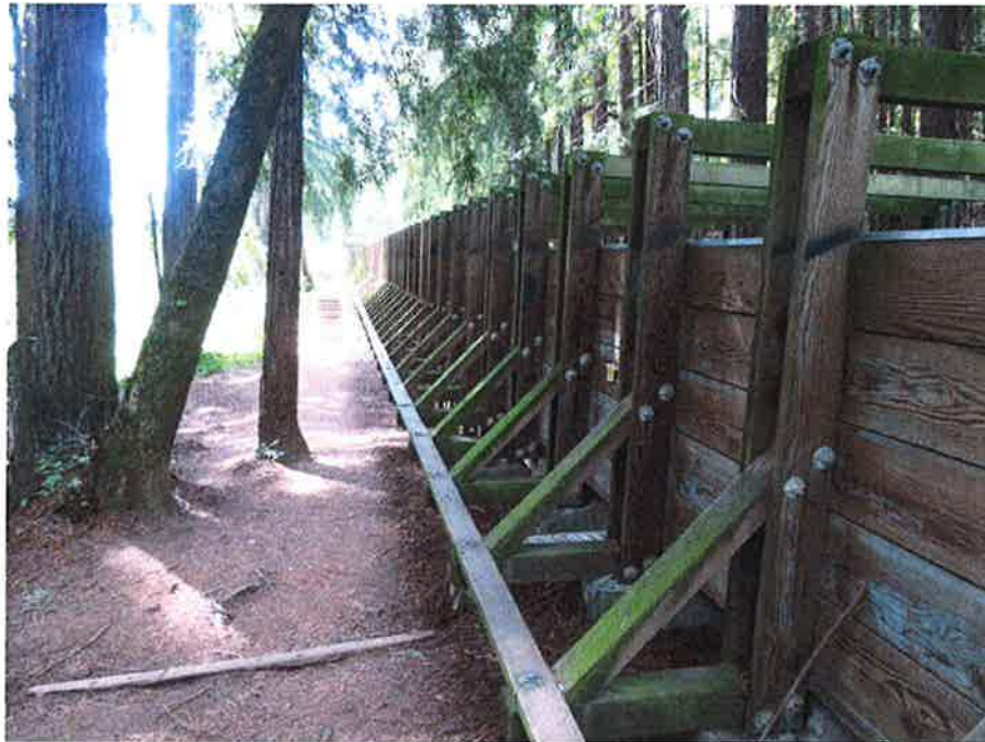
The right side of the wood timber spillway flume looking in the upstream direction. Pressure treated timbers supporting the flume appear to be in good condition, as does the stainless steel flume sheathing, the under flume supports, and flume foundation connections.
