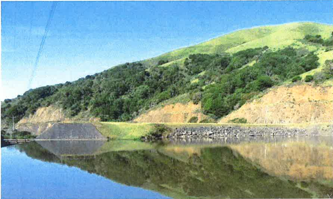
The upstream face as viewed from the upstream end of the spillway channel. The large boulder riprap face protection remains in good condition.
