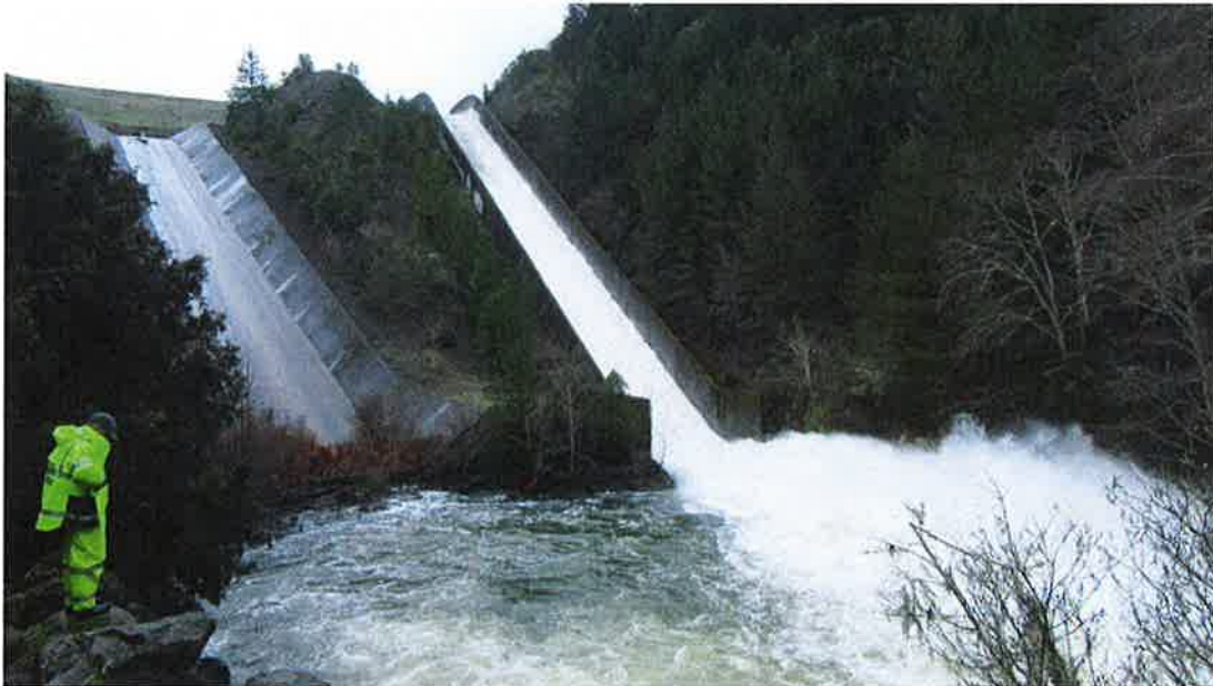
A large redwood log that has drifted into and was caught on the right side of the concrete spillway control weir requires removal, above. The photograph below shows flow within the concrete spillway channel entering the unlined spillway exit channel.
