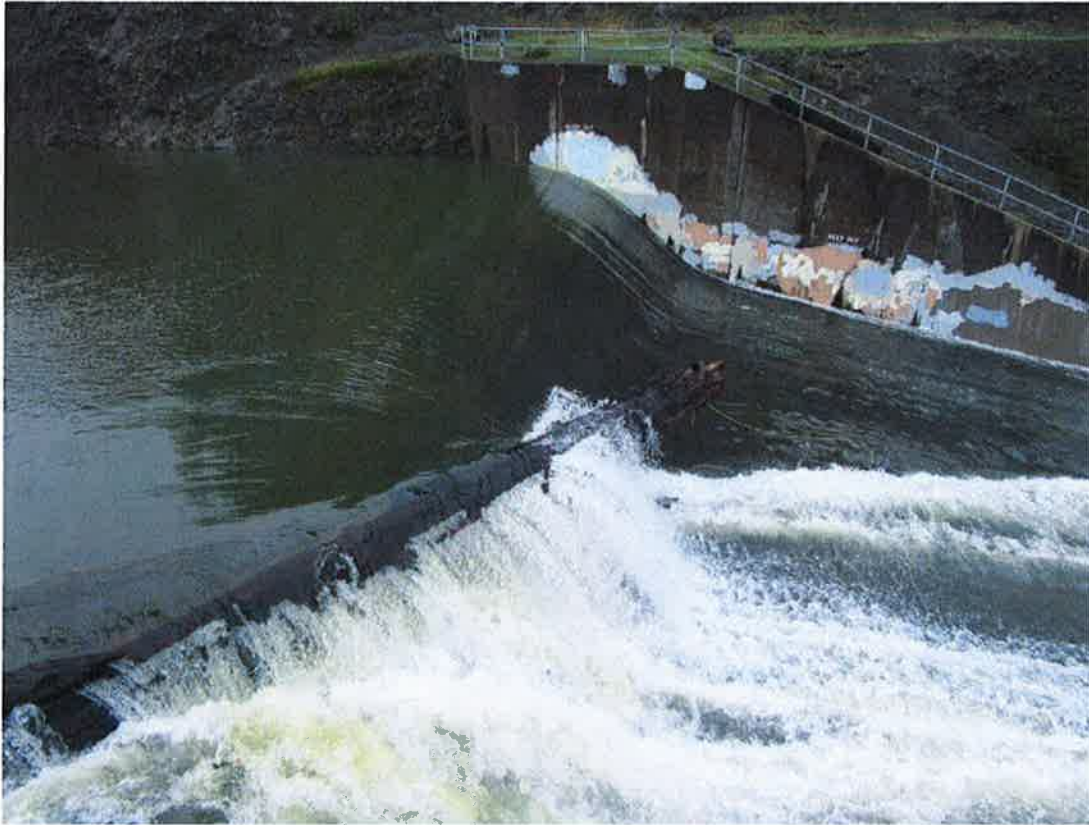
A large redwood log that has drifted into and was caught on the right side of the concrete spillway control weir requires removal, above. The photograph below shows flow within the concrete spillway channel entering the unlined spillway exit channel.
