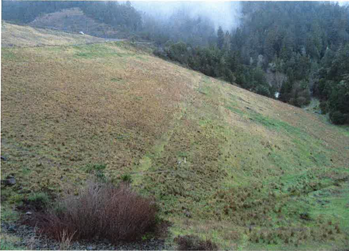
Looking across the downstream face of the embankment towards the left groin, above, and another look at the left groin and downstream toe, below. As evident by the photographs, vegetation control is excellent.
