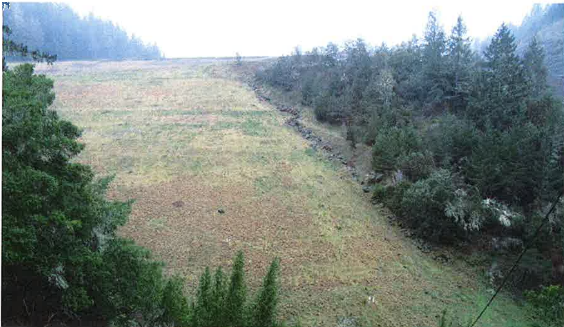
Looking across the downstream face of the embankment towards the left groin, above, and another look at the left groin and downstream toe, below. As evident by the photographs, vegetation control is excellent.
