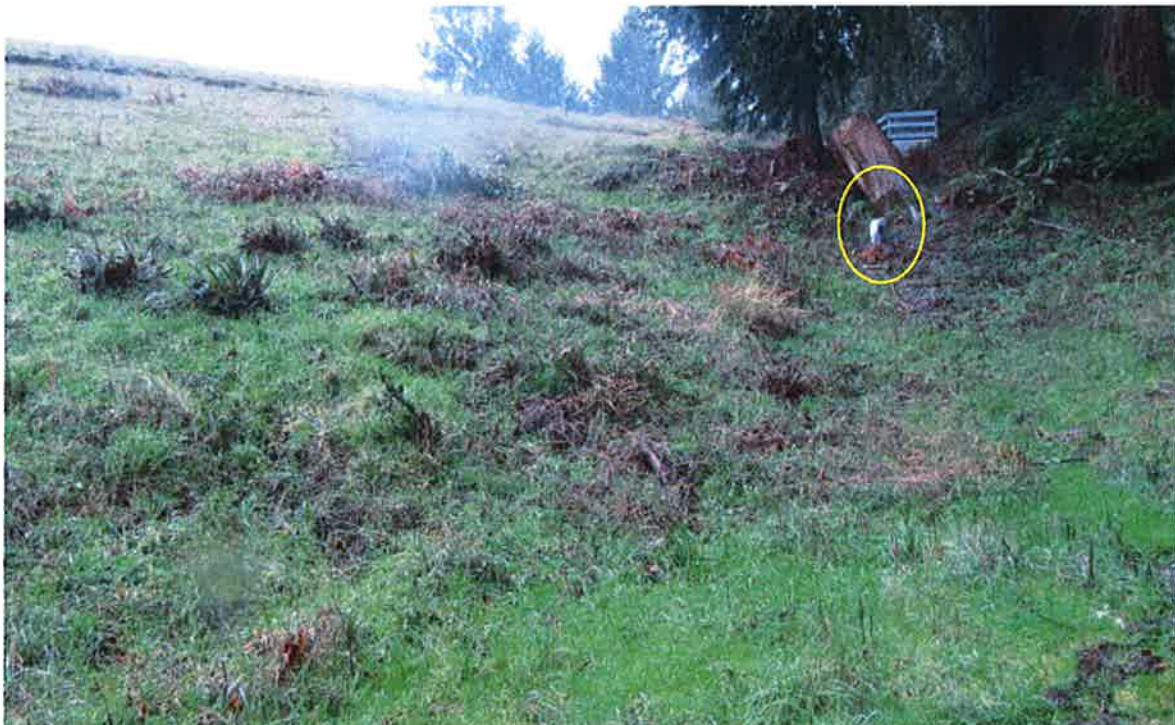
View towards the right downstream groin, above, and towards the left downstream groin, below. Note the location of the seepage collection pipe near the upper left groin (circled).
