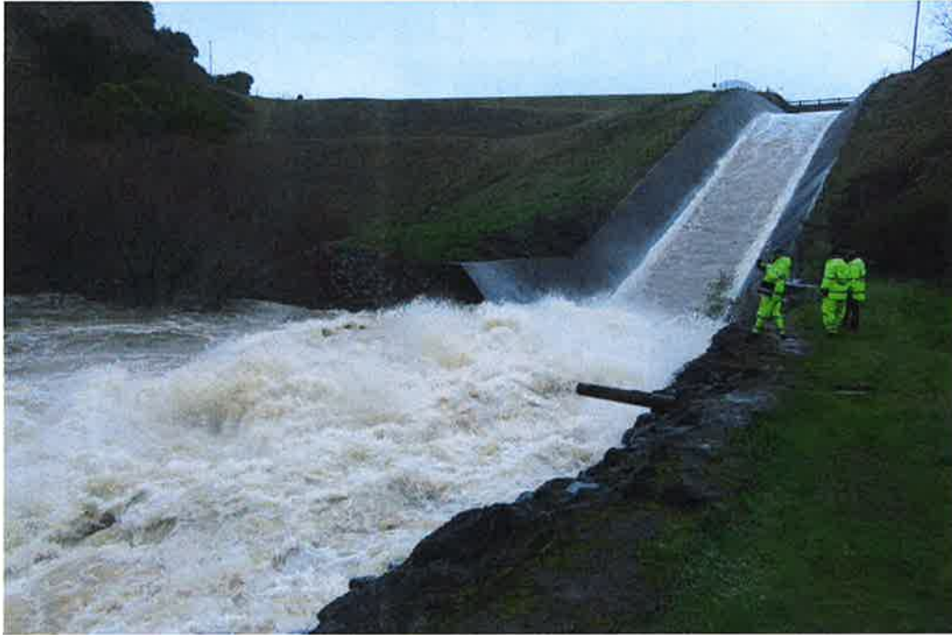
Spillway flow leaving the concrete spillway channel and entering the unlined exit channel, above. The bottom photograph shows the recently repaired downstream most outlet control valve. A recently installed and very well constructed guardrail installed to protect workers operating the downstream outlet control valves.
