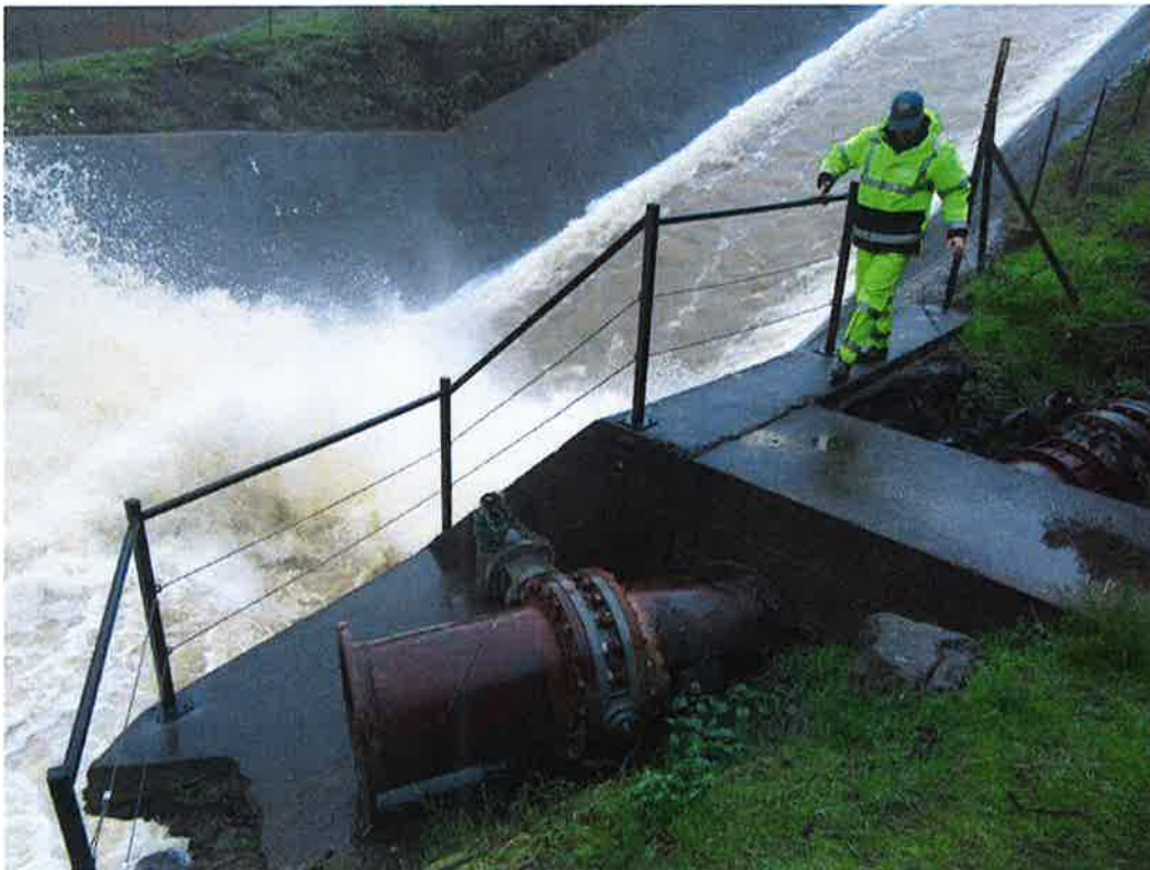
Spillway flow leaving the concrete spillway channel and entering the unlined exit channel, above. The bottom photograph shows the recently repaired downstream most outlet control valve. A recently installed and very well constructed guardrail installed to protect workers operating the downstream outlet control valves.
