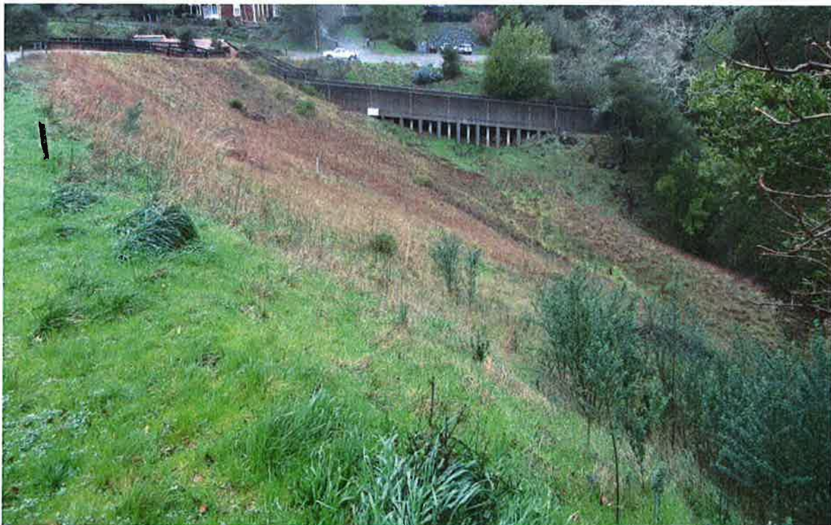
View towards the right downstream groin, above, and towards the left downstream groin and spillway, below. Emerging bushes scattered throughout the downstream face should be removed later in the season.
