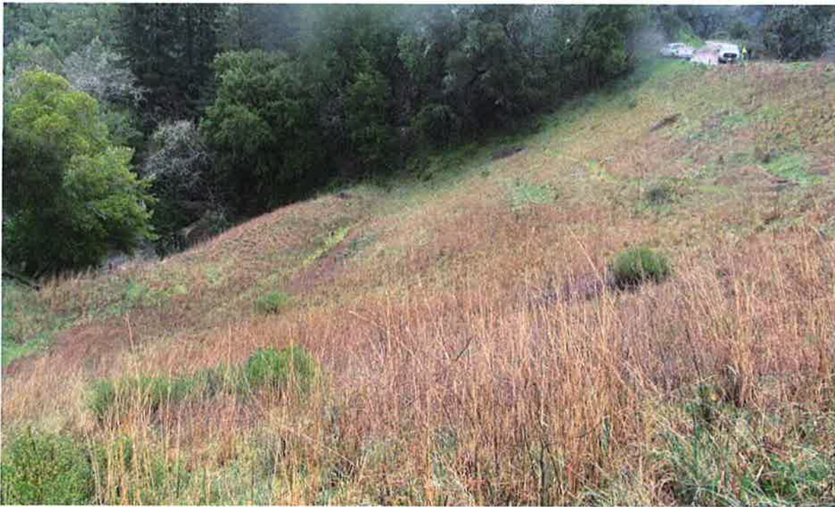
View towards the right downstream groin, above, and towards the left downstream groin and spillway, below. Emerging bushes scattered throughout the downstream face should be removed later in the season.
