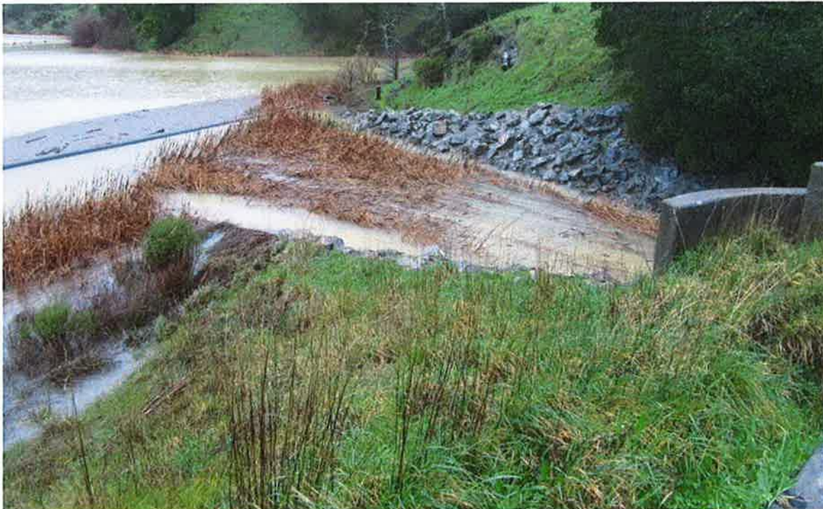
The upstream face looking towards the spillway entrance (indicated), above. A closer look at the spillway entrance, and the polyethylene log boom protecting the entrance, is shown below.
