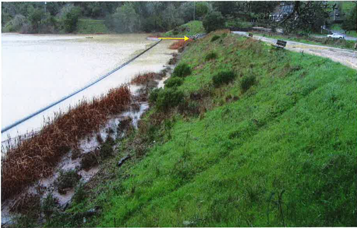
The upstream face looking towards the spillway entrance (indicated), above. A closer look at the spillway entrance, and the polyethylene log boom protecting the entrance, is shown below.
