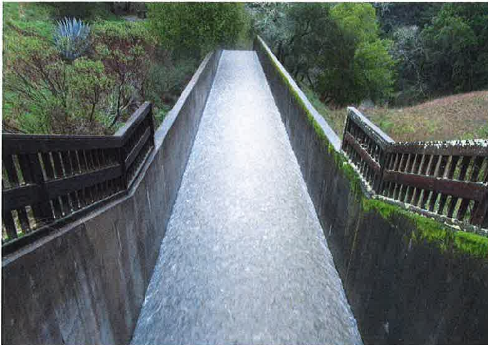
Flow through the concrete spillway channel appears normal, above.
