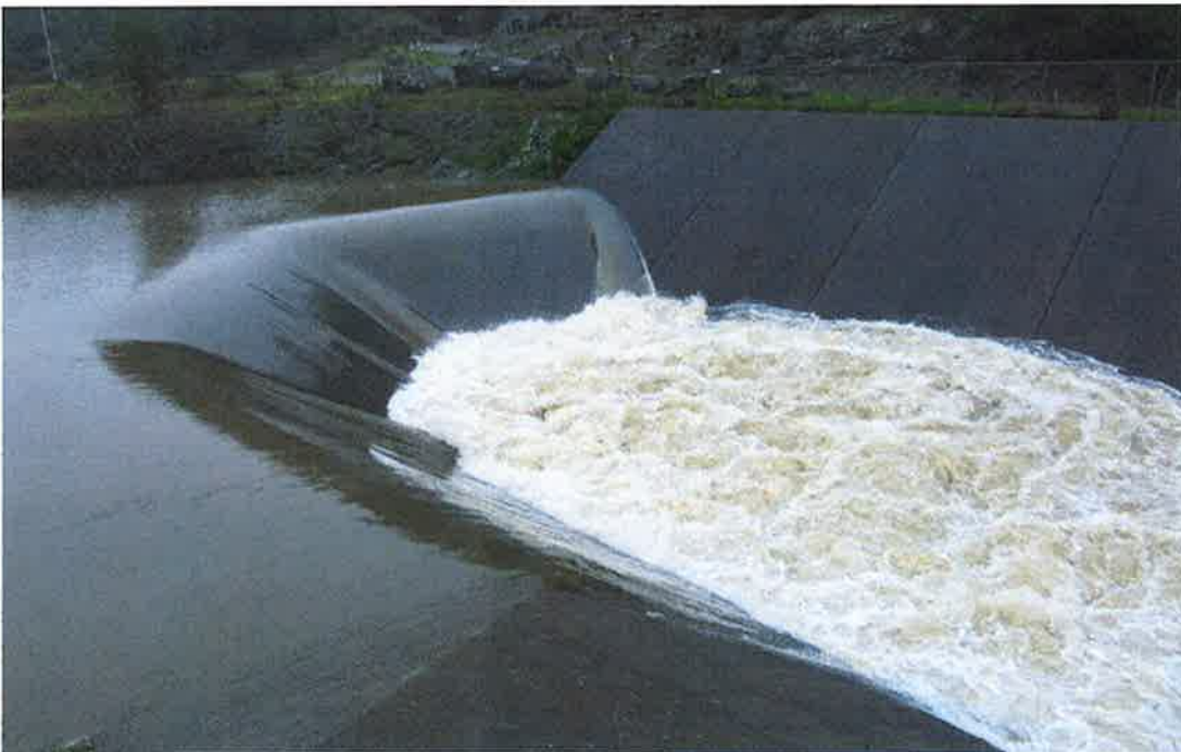
1.3' flow over the spillway entrance weir.
