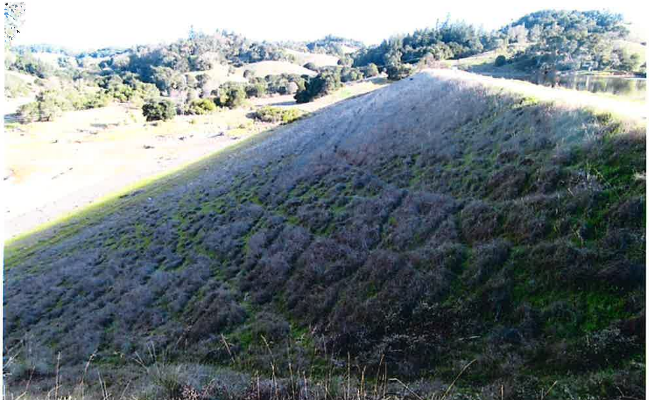
The downstream face looking towards the left abutment, above, and looking towards the right abutment, below. Vegetation control is very good.
