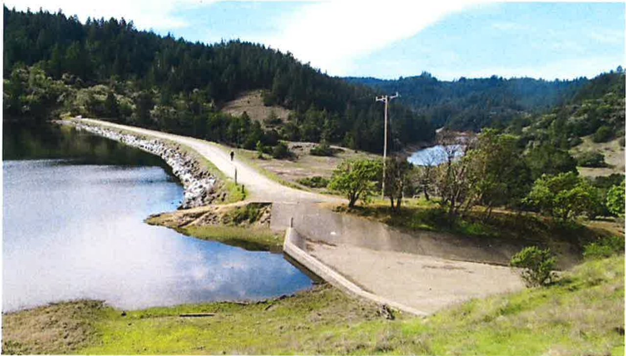
The upstream face and spillway entrance as viewed from the right abutment. The recently placed large boulder riprap along the upstream face waterline is lighter in color than the original rock.
