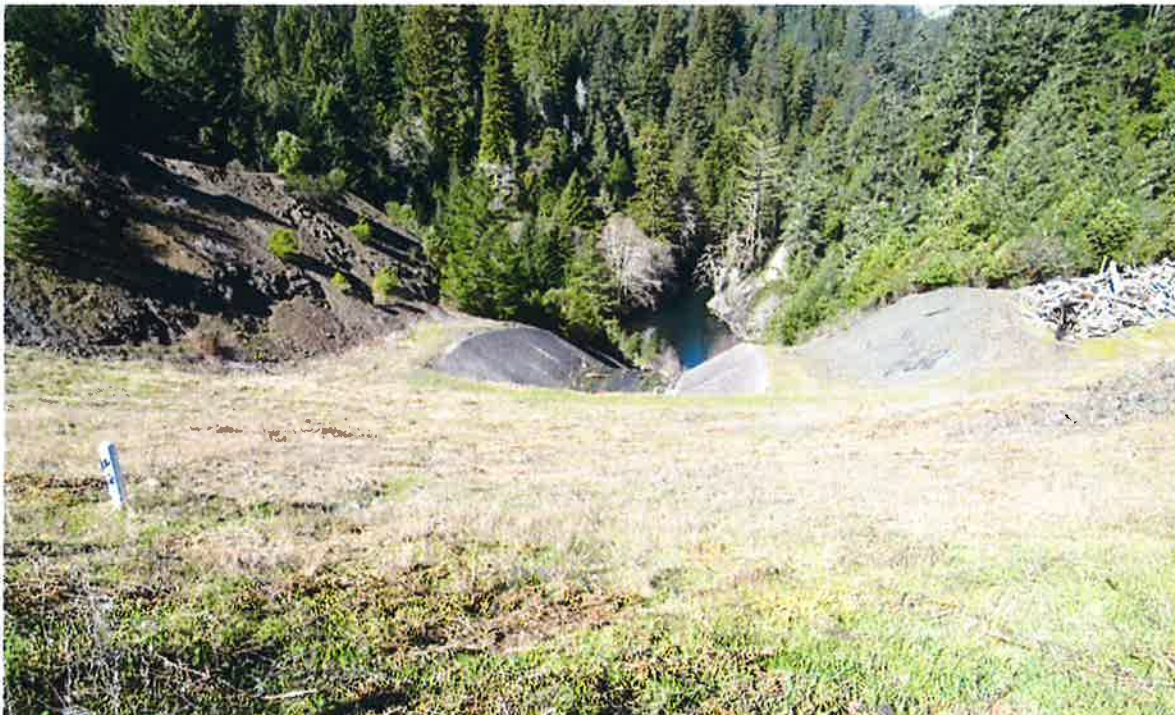
The downstream face of the main portion of the embankment, above, and the downstream face of the embankment above the original spillway, below. Vegetation control remains excellent.
