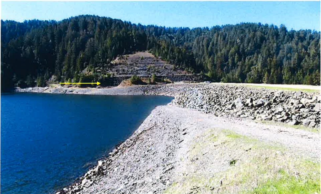
The upstream face looking towards the spillway entrance (indicated by arrow), above, and looking towards the right abutment, below.
