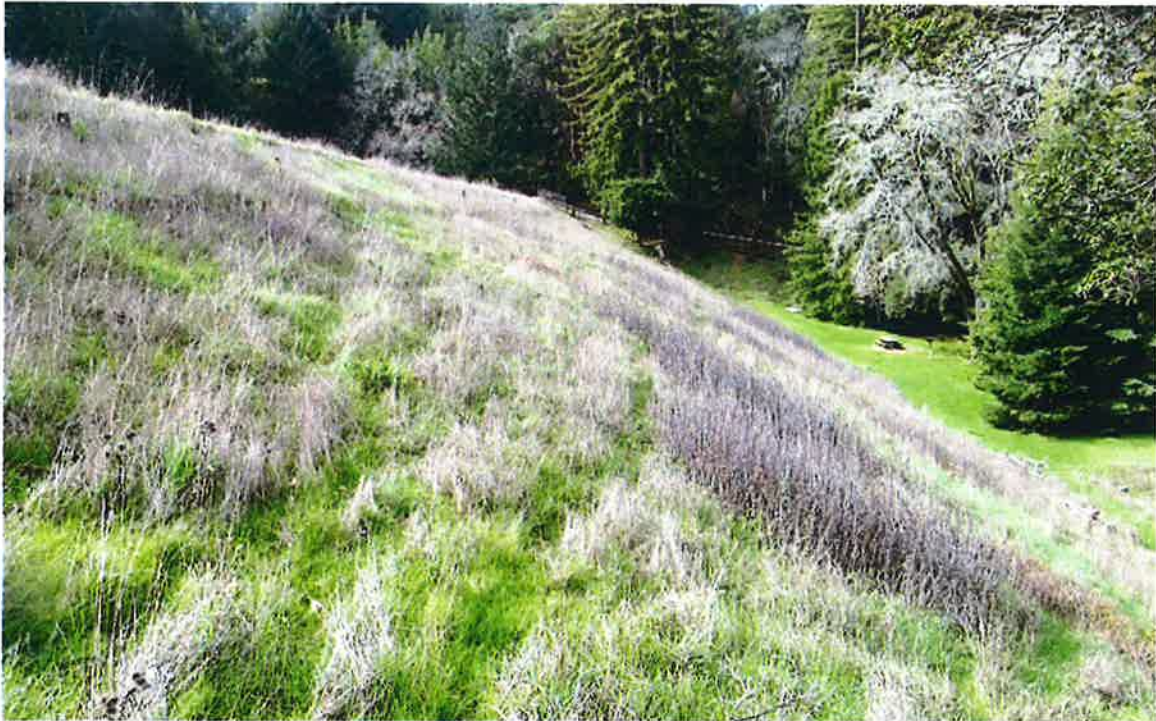
The downstream face looking towards the left abutment, above, and looking towards the right abutment, below. Vegetation control along the downstream face is quite good.
