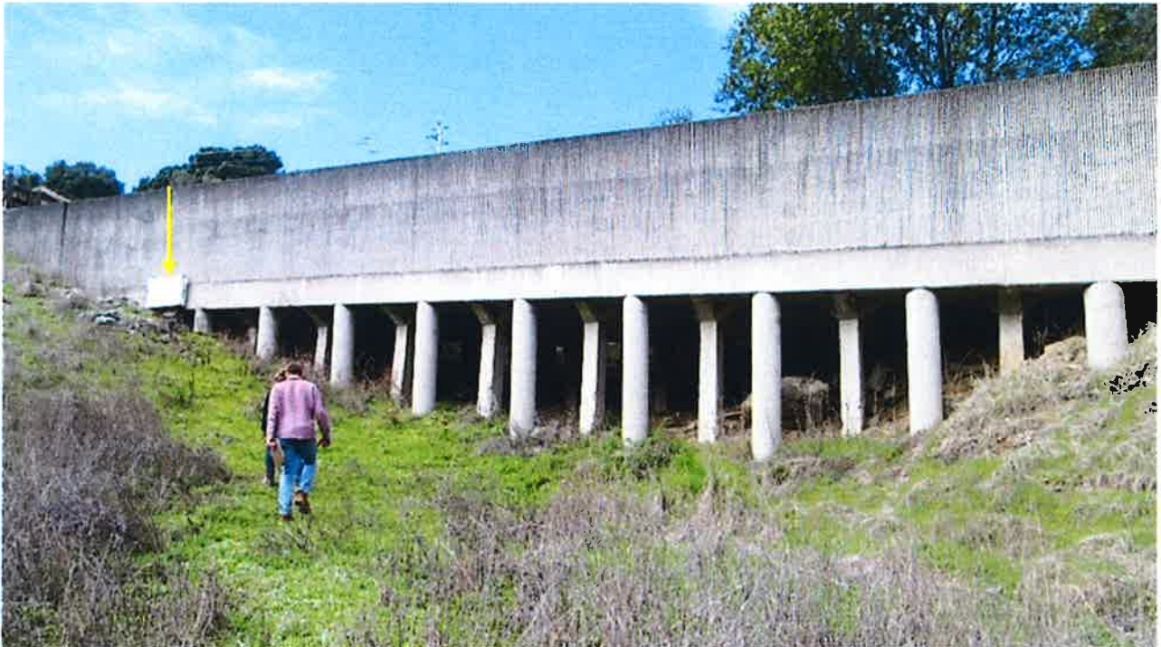
Looking across the downstream face towards the raised spillway section, above, with a closer look at the raised spillway below. The location of the crack within the spillway is indicated in both photographs.
