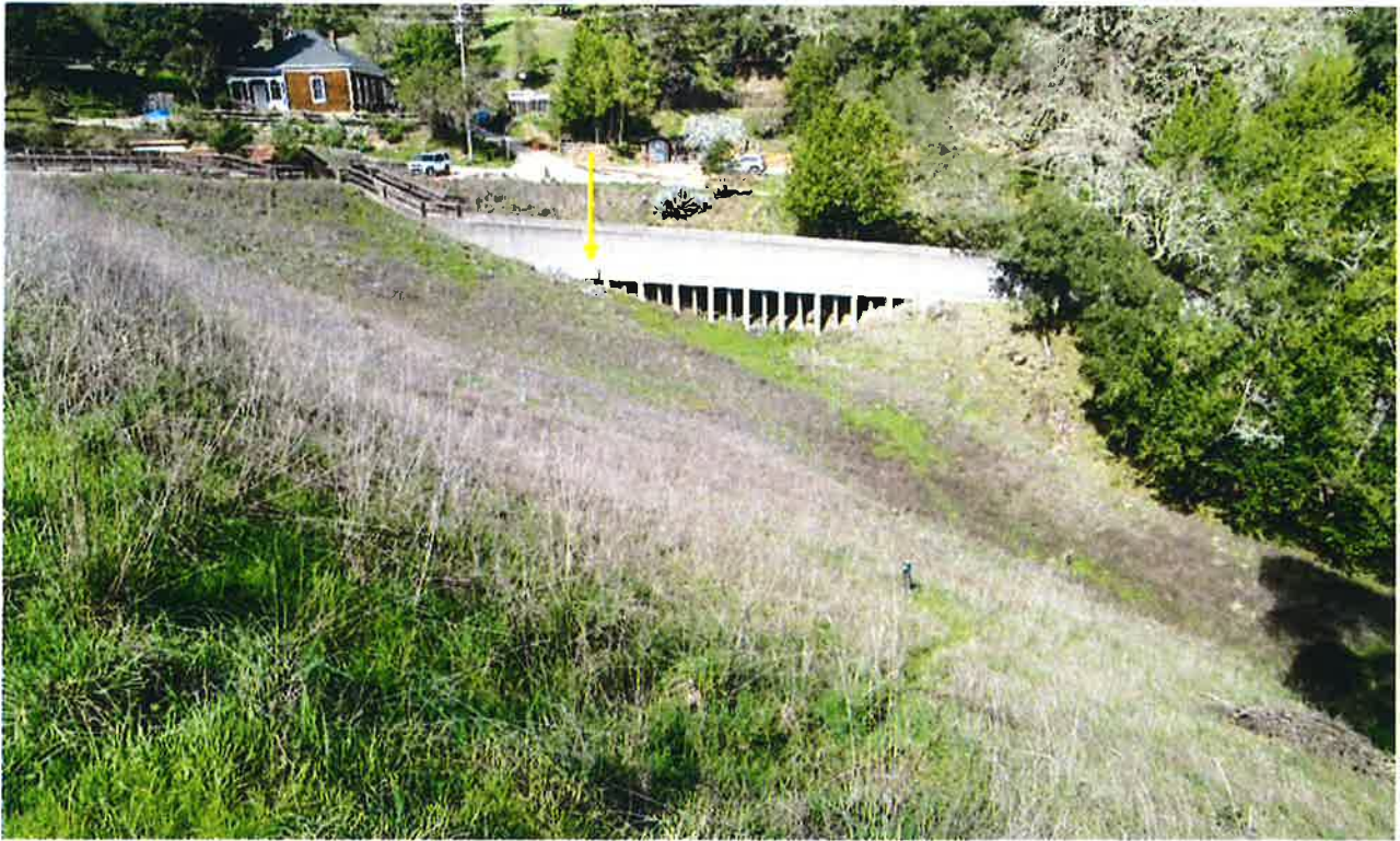
Looking across the downstream face towards the raised spillway section, above, with a closer look at the raised spillway below. The location of the crack within the spillway is indicated in both photographs.
