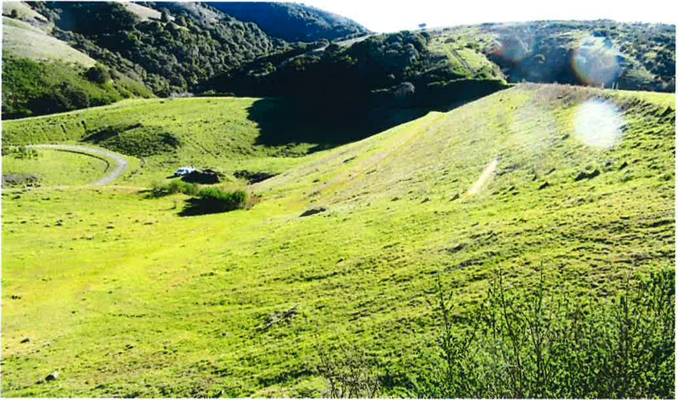
The downstream face as viewed from the right spillway abutment, above, and as viewed from the alternative access road along the right side of the dam, below. Vegetation control is excellent.
