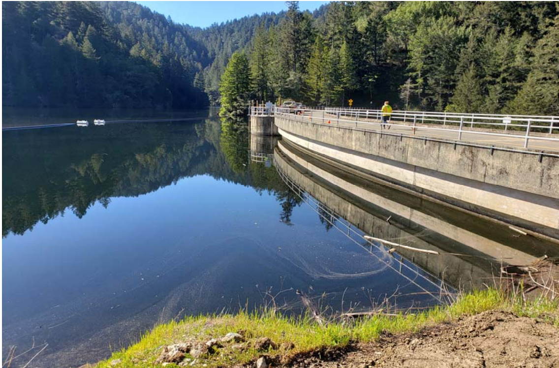
Photo 1: View of the upstream face as seen from the right abutment.
