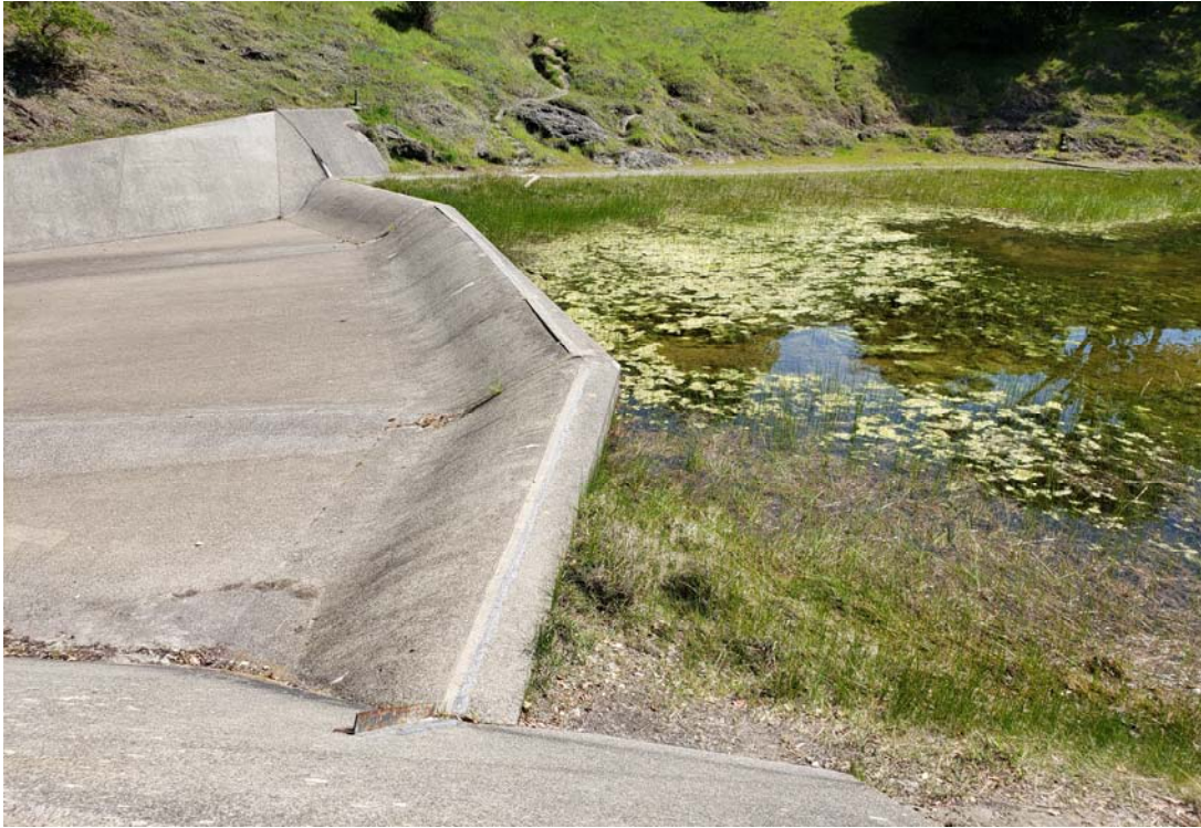
Photo 3: View of the spillway approach and concrete weir.
