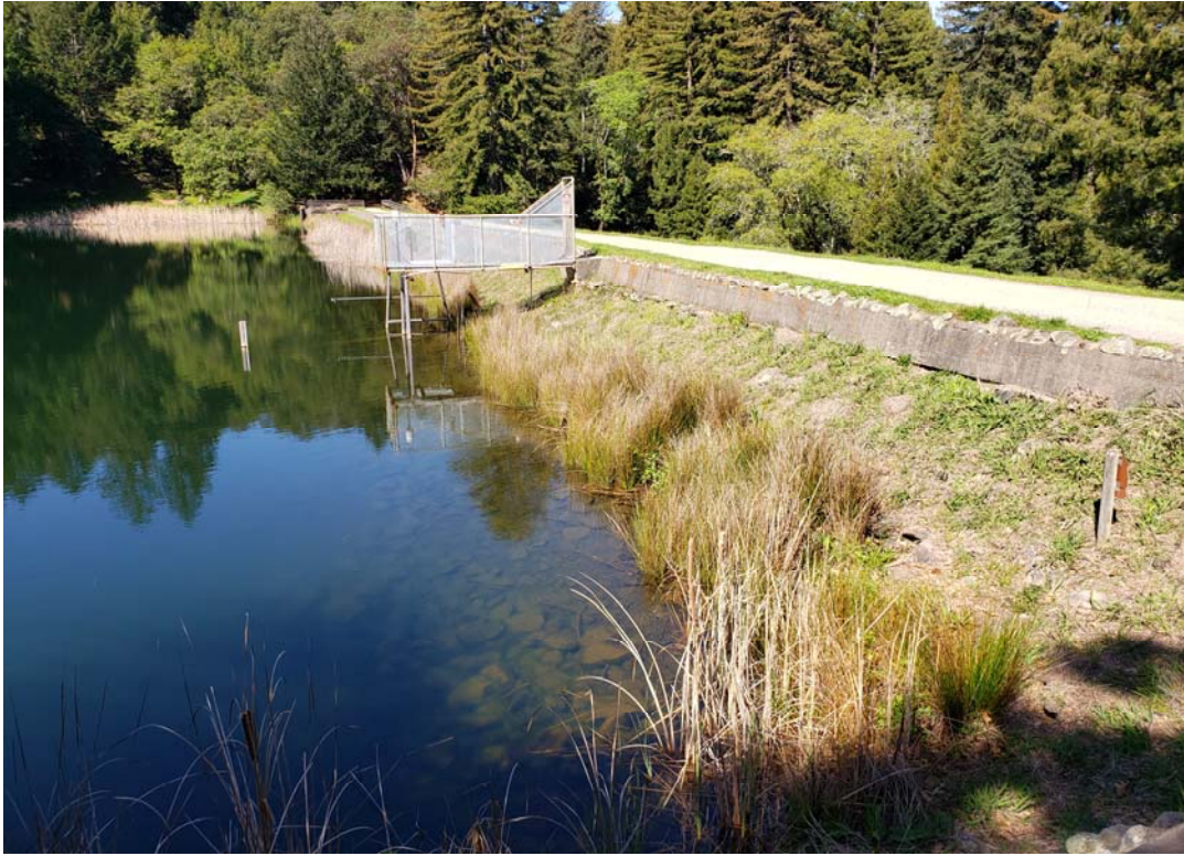
Photo 1: View of the upstream face as seen from the right abutment.
