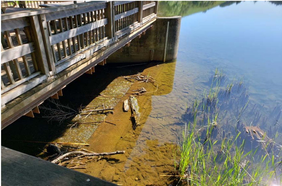
Photo 4: The spillway approach was clear and unobstructed and slightly spilling.
