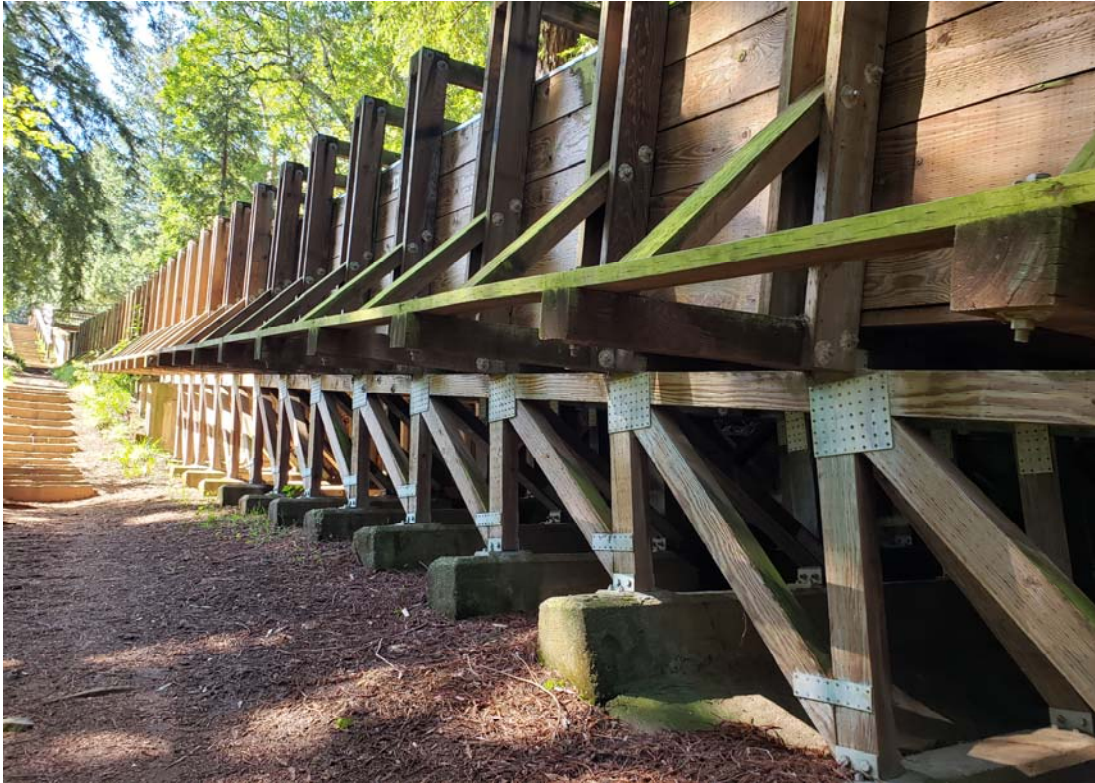
Photo 3: View of the timber supported flume, looking upstream.
