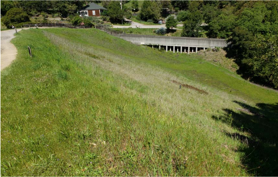
Photo 1: View of the downstream face as seen from the right abutment.
