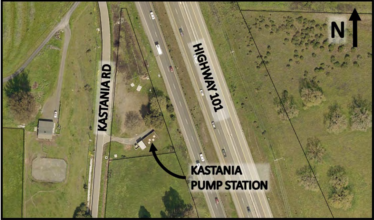
Exhibit A: Kastania Pump Station, 4100 Kastania Road, Petaluma
